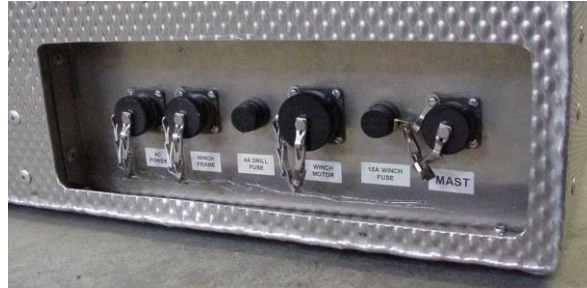
Figure 12 – Control Panel Back Panel
